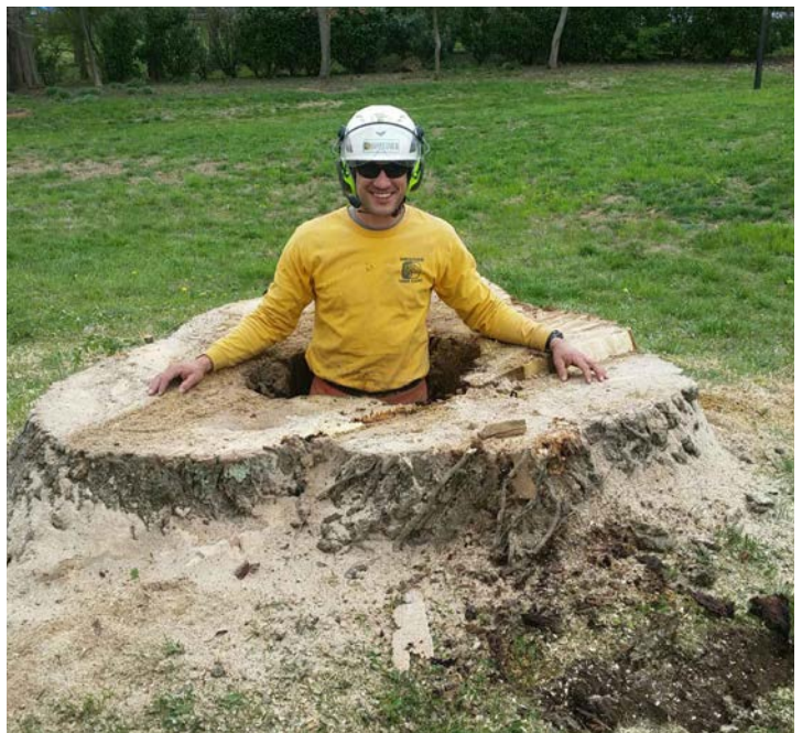
Often times decay is not always visible to the naked eye. The resistograph showed that this tree was rotting from the inside out.
