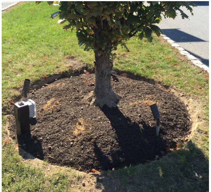
After removing excess soil and mulch, this Oak's root flare is now properly exposed.
